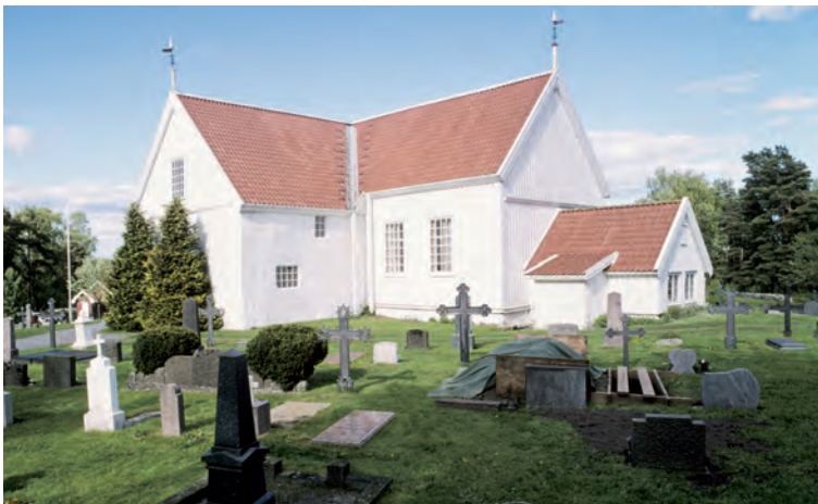
Fig. 40 The medieval stone church of Tromøy, Aust-Agder. (Photo: Christer Westerdahl, 2004)
